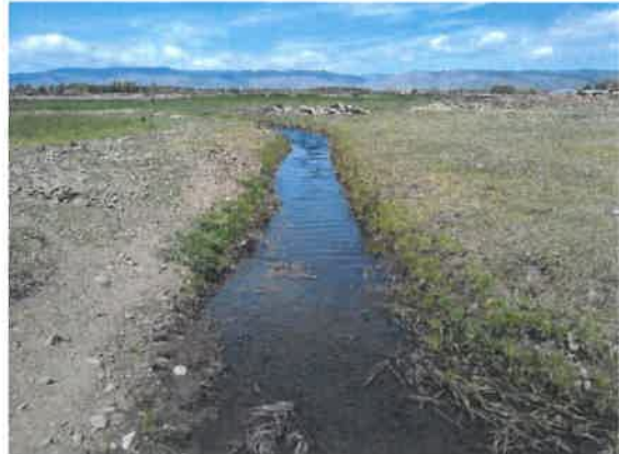
Typical irrigation ditch.
